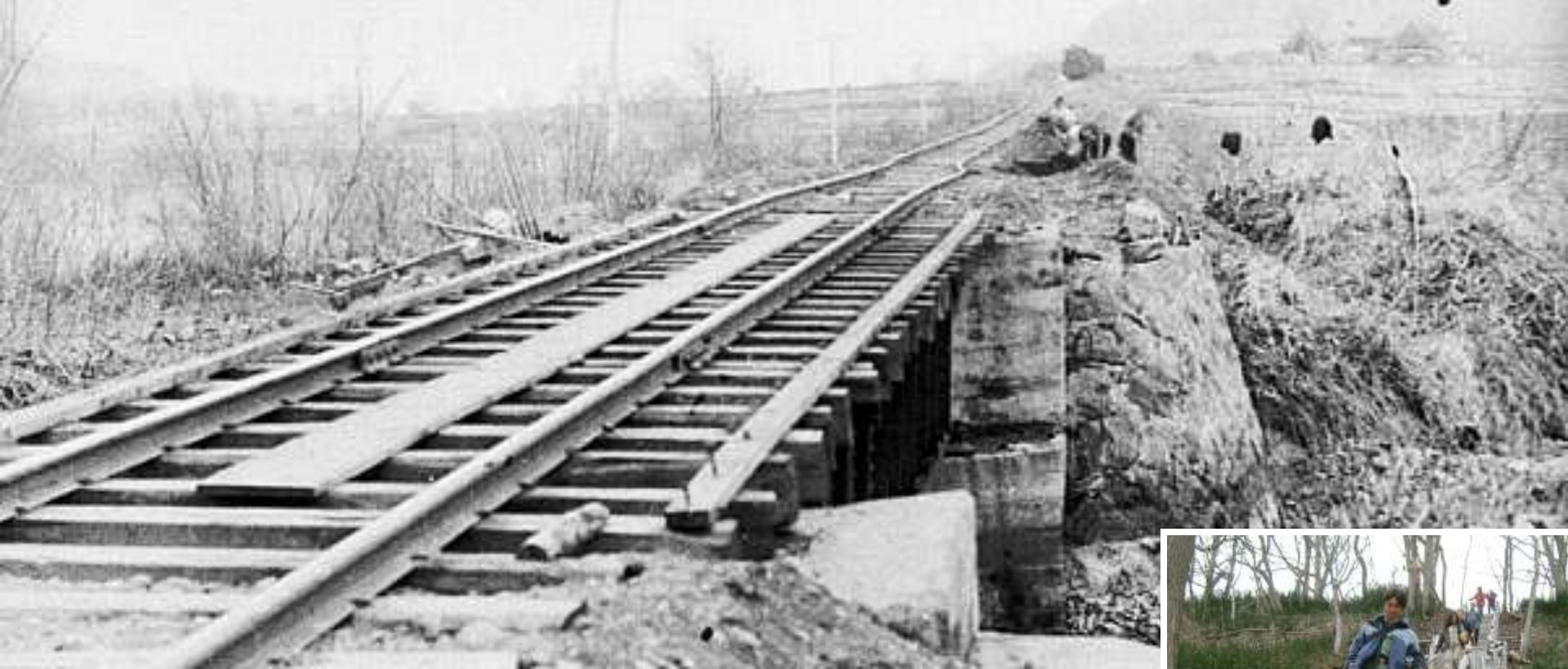
The pier of National Railway was raised up about 30m high.
