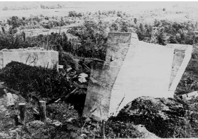
The pier of National Railway was raised up about 30m high.
